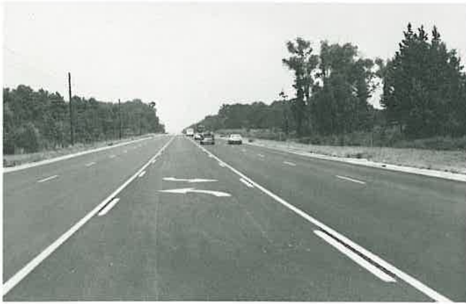
New construction of U.S. 71 five-lane section north of Texarkana.
