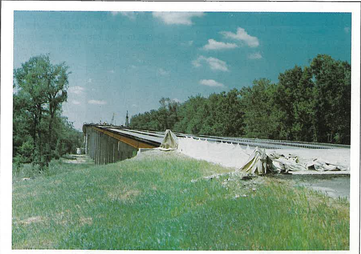
St. Charles White River Bridge under construction on State Highway 1.
