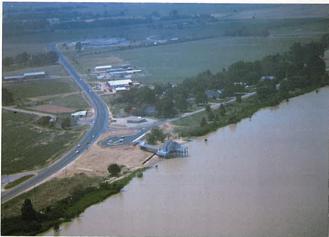
U.S. Highway 65 at Lake Village looking north.
