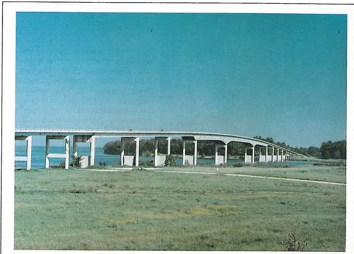
Pendleton Bridge over the Arkansas River on U.S. Highway 165.
